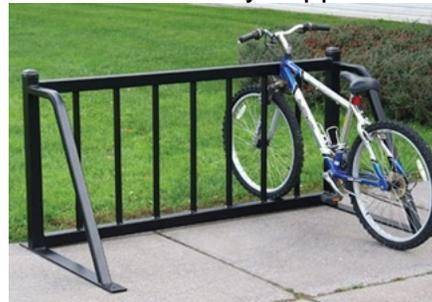
Wheel-bender racks do not support the bike in two places and when the bike falls over it ruins the wheel.
